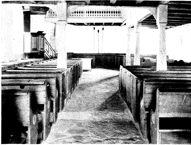
Looking from West Entrance, Showing Timbers Under Gallery Floor, Collection Bags on Front Wall, and Imported Pulpit of European Red Walnut.
