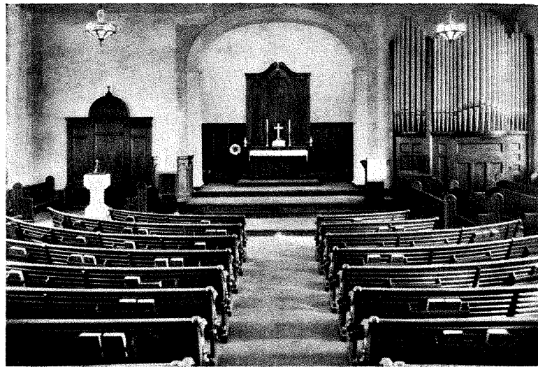
Interior of Present Church Renovated 1930.
